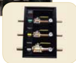
Zone valve boxes
